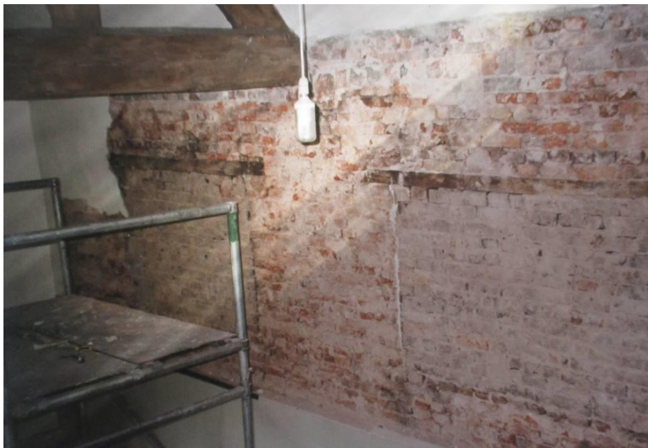
Figure 3: Internal works reveal former window openings (Stourbridge MH Archive)
